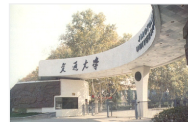
External wall insulation system Vocational Education Center Shanghai Jiao Tong University
