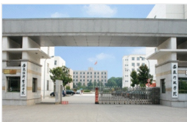
External wall insulation system project Party School of the CPC Committee, Anhui province, Hefei
