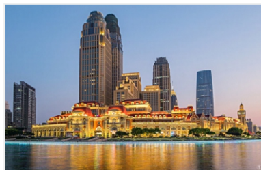
Tianjin Jinwan Square external wall insulation system project
